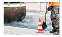
9. The Cecabase RT<sup>®</sup> additive is used to fluidize road bitumen when it is laid. The bitumen is therefore heated to a lower temperature, reducing energy consumption by:
